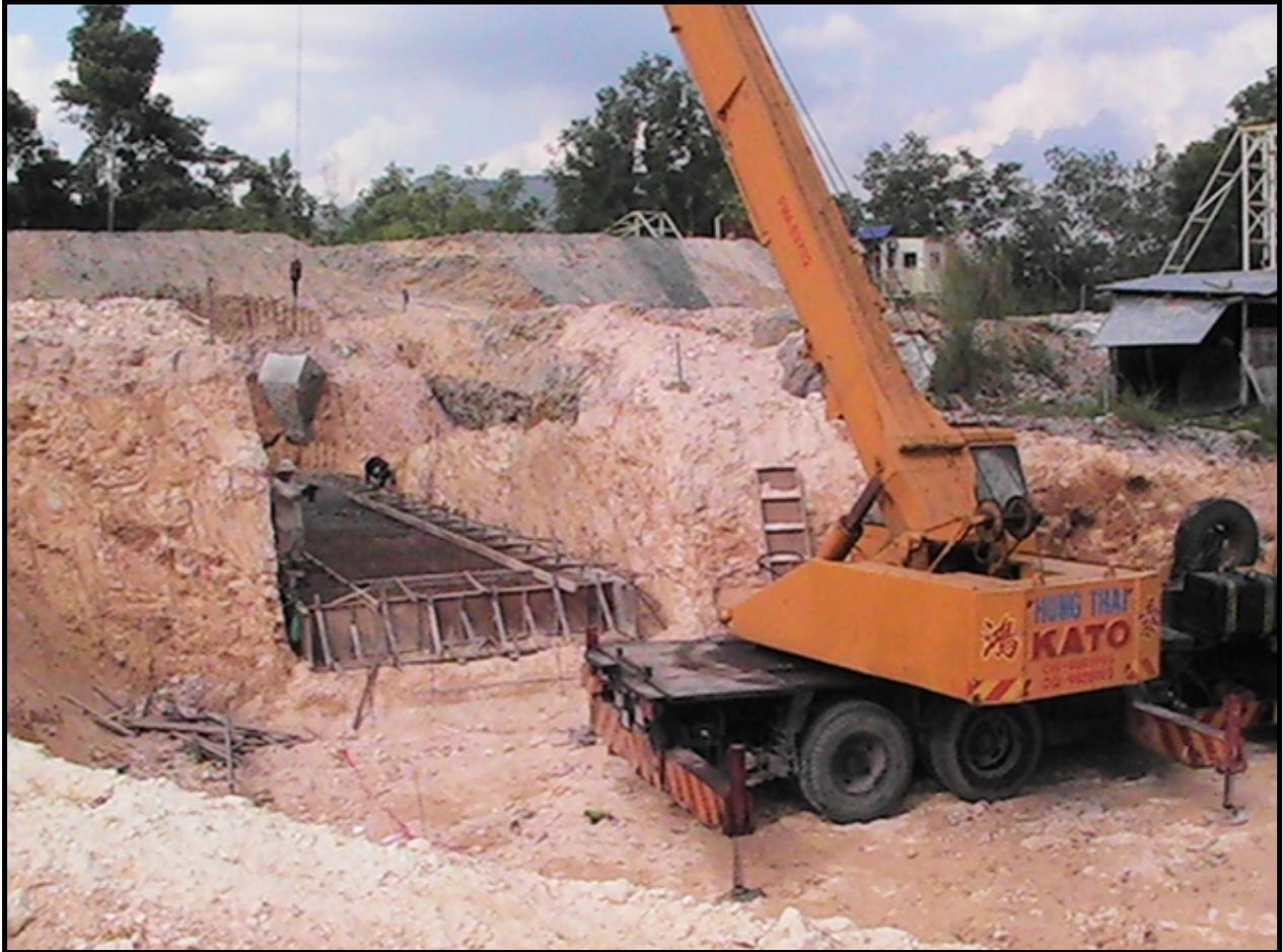
Recent pouring of concrete for the base of the reclaim tunnel at Bukit Ibam
