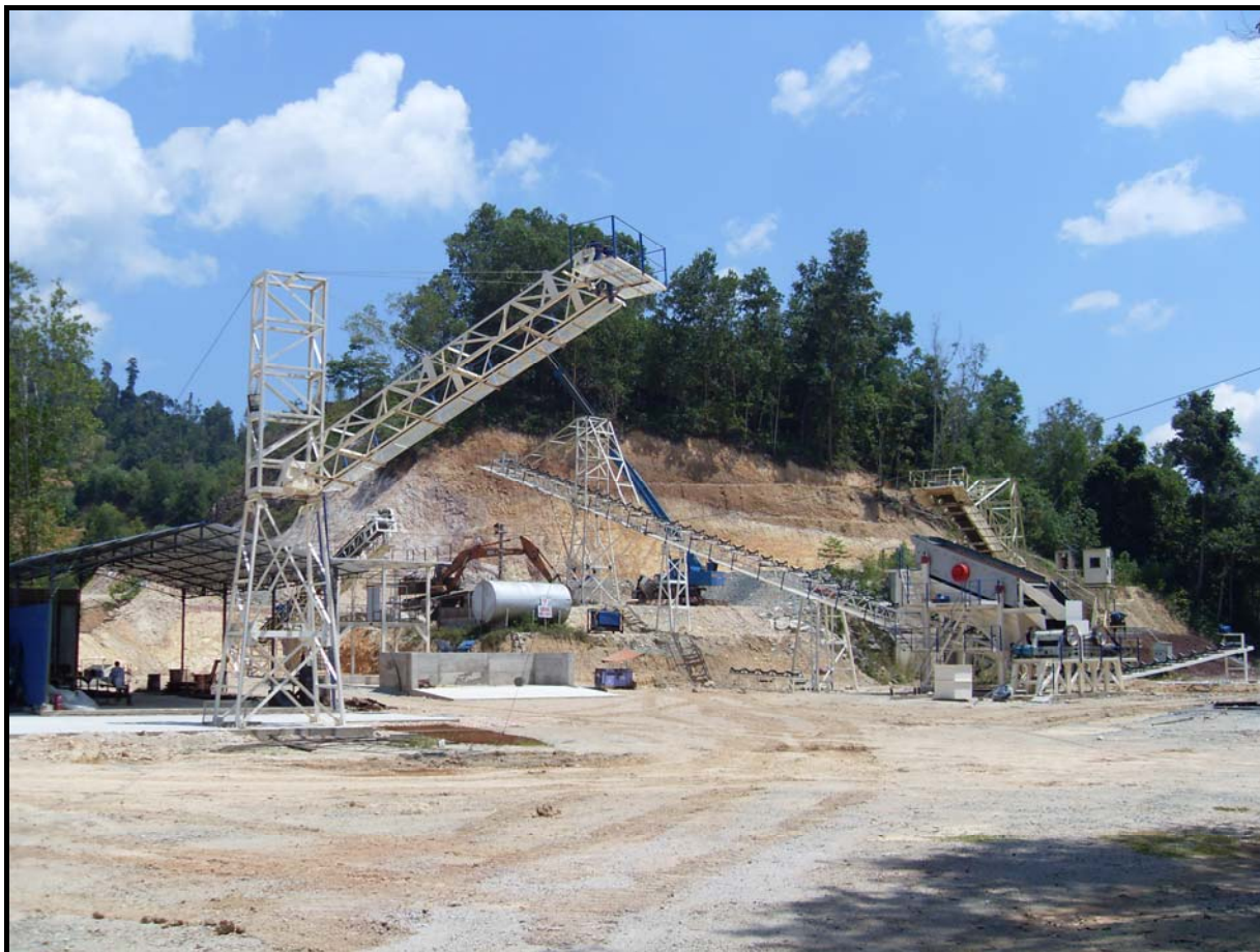
Figure 3: Construction activity at the Bukit Ibam processing plant site.
